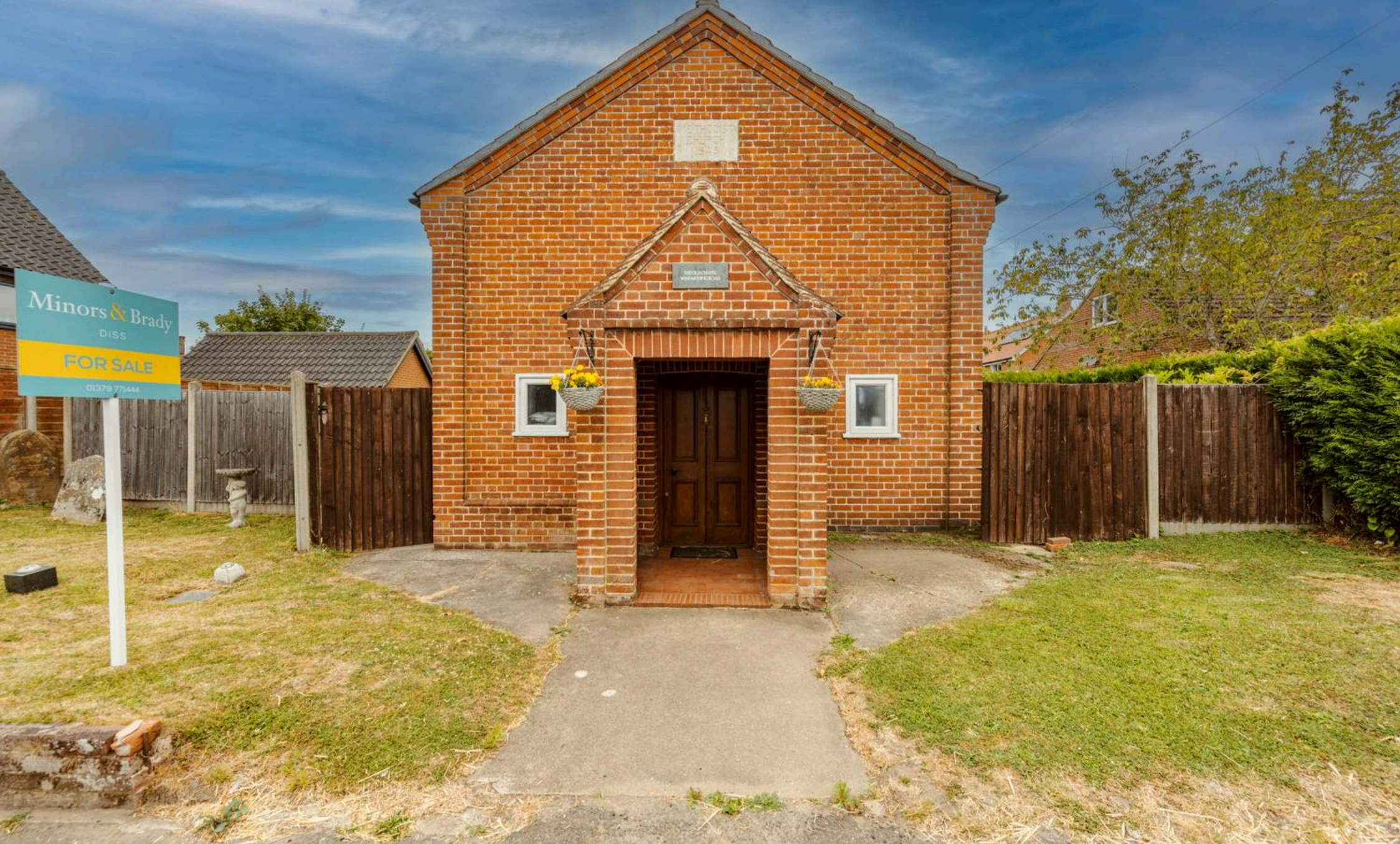
The Old Chapel Winfarthing Road, Shelfanger Minors & Brady
