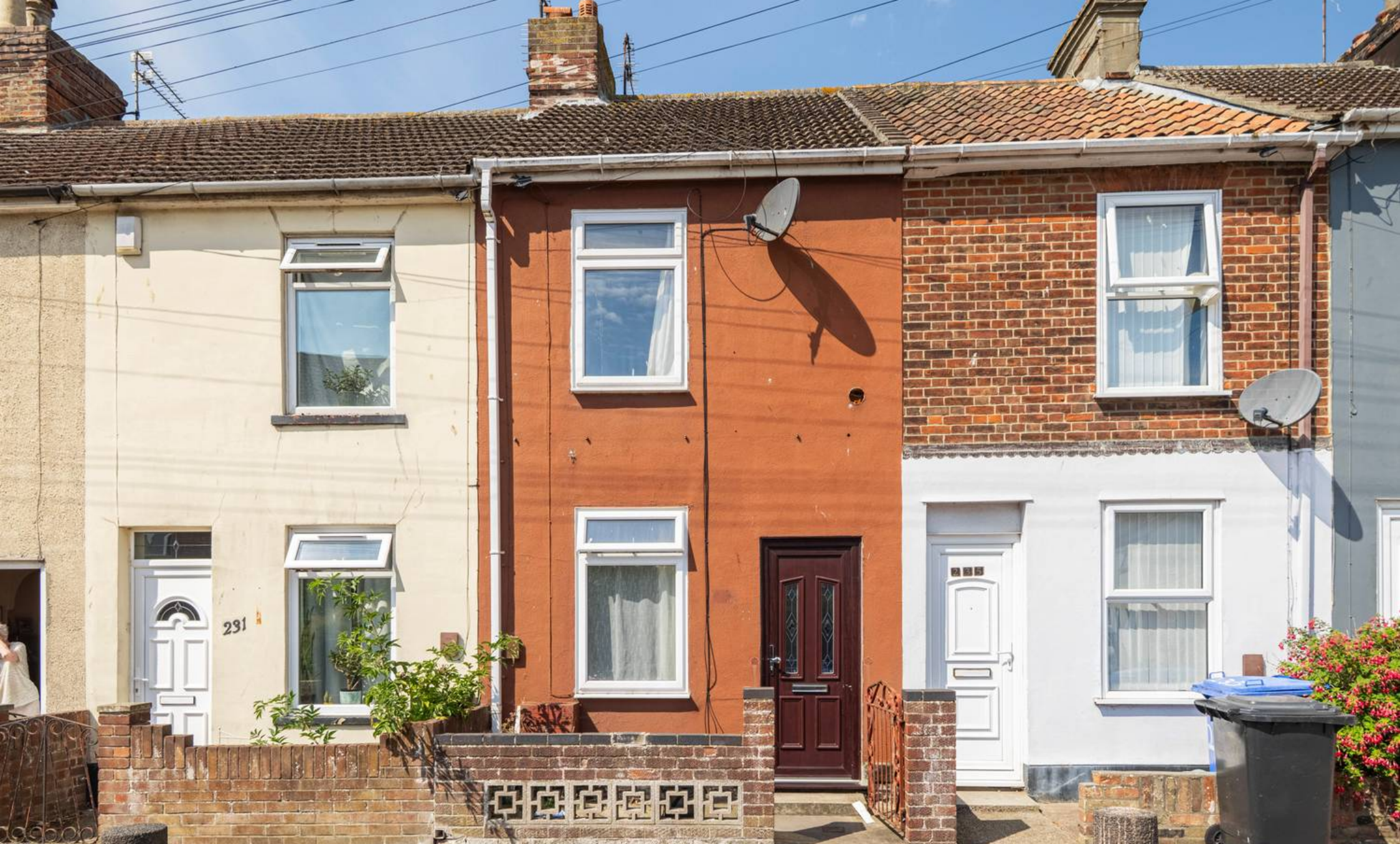
233 Raglan Street, Lowestoft
