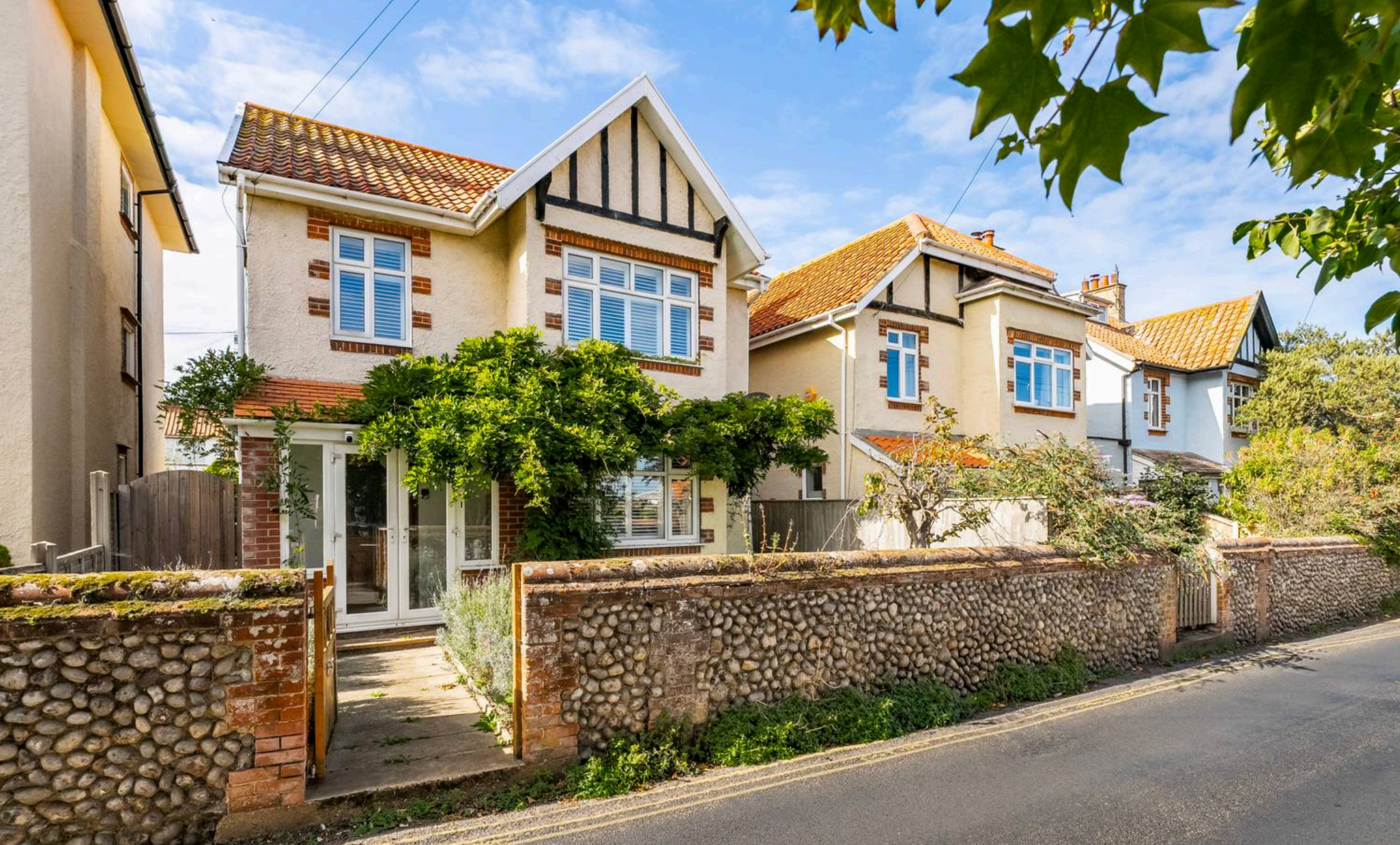
Cherry Tree Cottage Water Lane, West Runton
